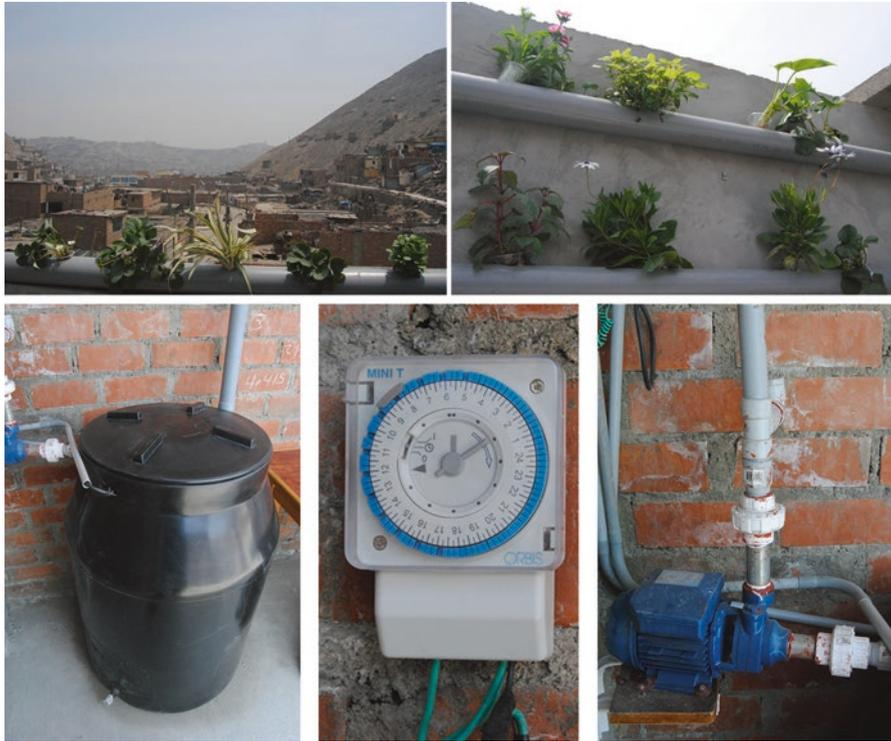
**Fig. 2** Modified NFT system that works with a pump in the children playhouse at Monterrey, Lima, Peru (Photo: F. Orsini). *Top*, views of the hydroponic gardens, *bottom, left to right*, tank for the nutrient solution, electric timer and hydraulic pump
