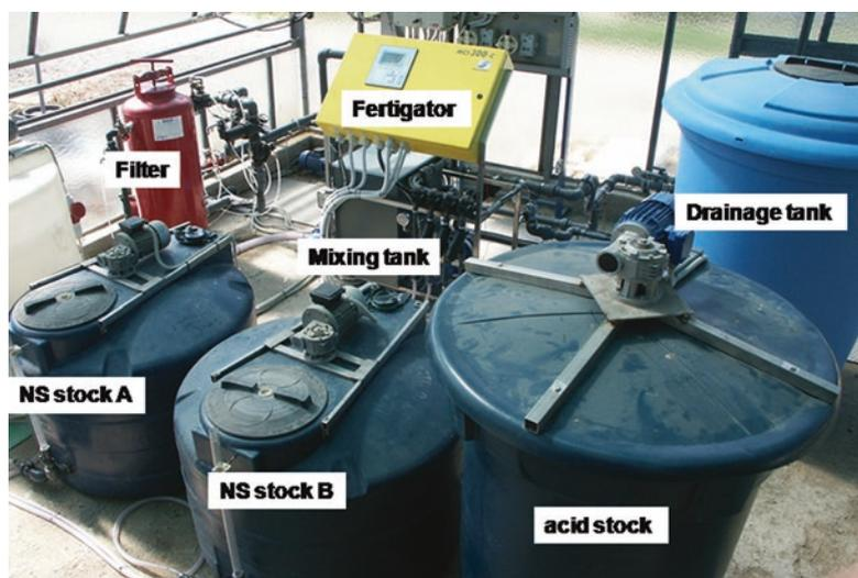
**Fig. 2** An example of a medium-tech fertigation system. Two stock nutrient solutions and diluted acid are mixed to raw water with Venturi injectors under the control provided by EC and pH probes. The controller also schedules irrigation based on weather-based estimation of crop evapotranspiration
